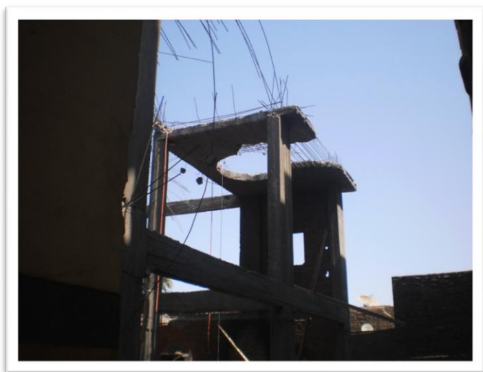
A dome demolished by Christians.
